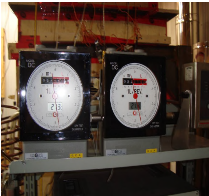
Picture 11: Dry gas meter
